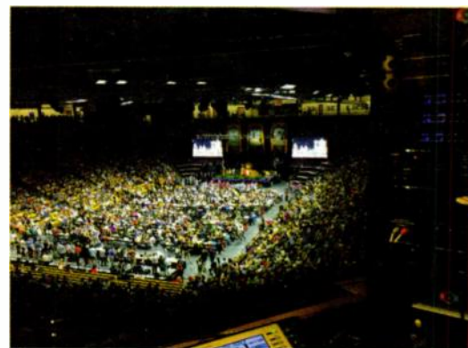
The Coors Events Center now sports a Bose Professional RoomMatch DeltaQ speaker system.
