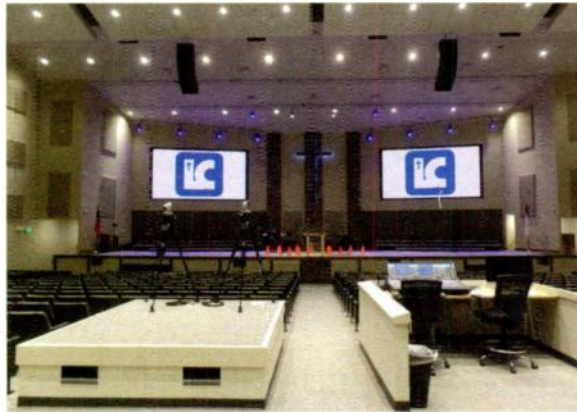
Inside The Lamb's Chapel's new sanctuary, an audio system based on RCF HDL20-A line array modules and an Allen & Heath dLive S5000 console ensures that each of the 2,000-plus congregants can hear every word.
