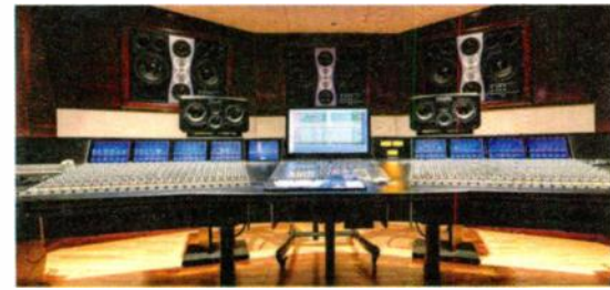
B Pro Production’s Studio A houses a 48-channel SSL Duality Delta Pro Station console.
