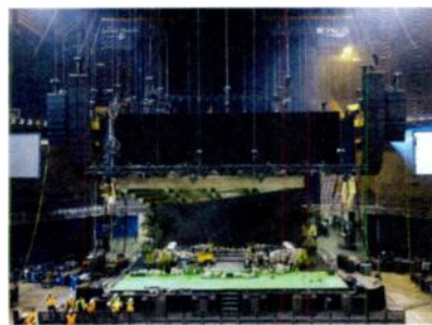
L-Acoustics’ K1-SB arrays (far left and right) were used to minimize LF intensity on the stage.
