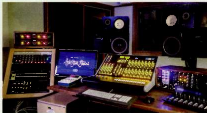
The control room at Hyde Street’s Annex, Rancho Rivera, is centered around a new API The Box console.
