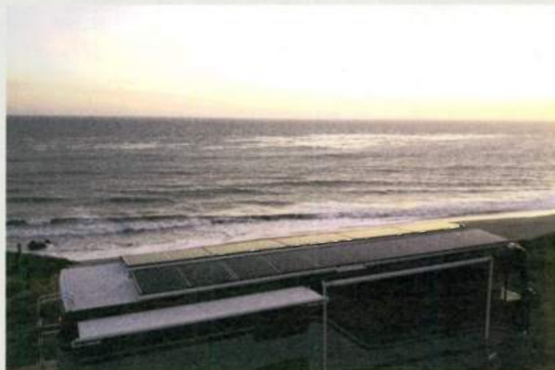
The solar panels generate enough electricity to power everything from air conditioners and the microwave to a four-piece rock band.
