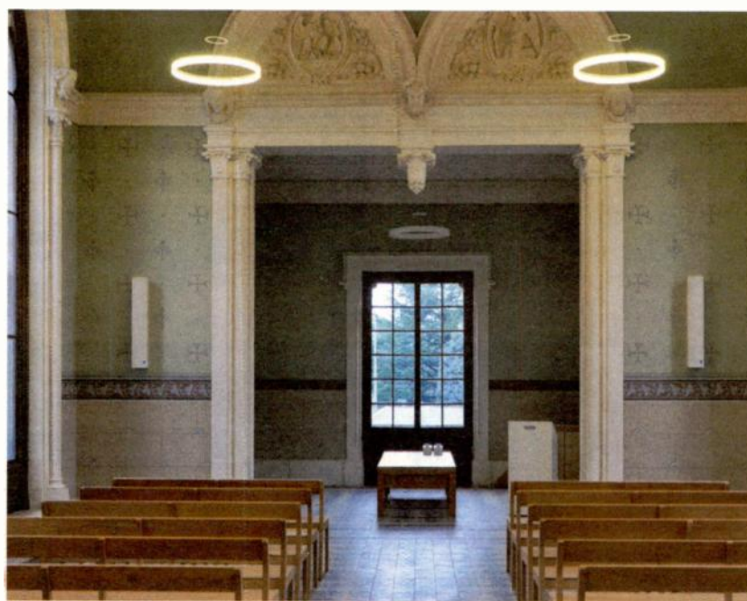
A 19th century Swiss chapel recently got a new Renkus-Heinz Iconyx system to help tame its aggressive reverberation.
