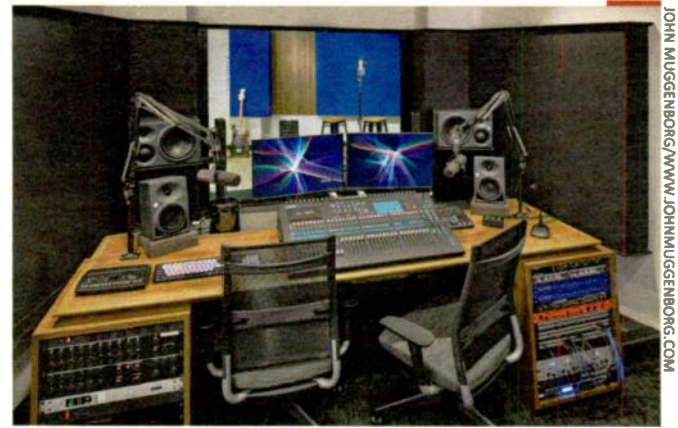
All the recording facilities in Stitcher's new headquarters, including Studio A's control room seen here, were designed by Walters-Storyk Design Group.
