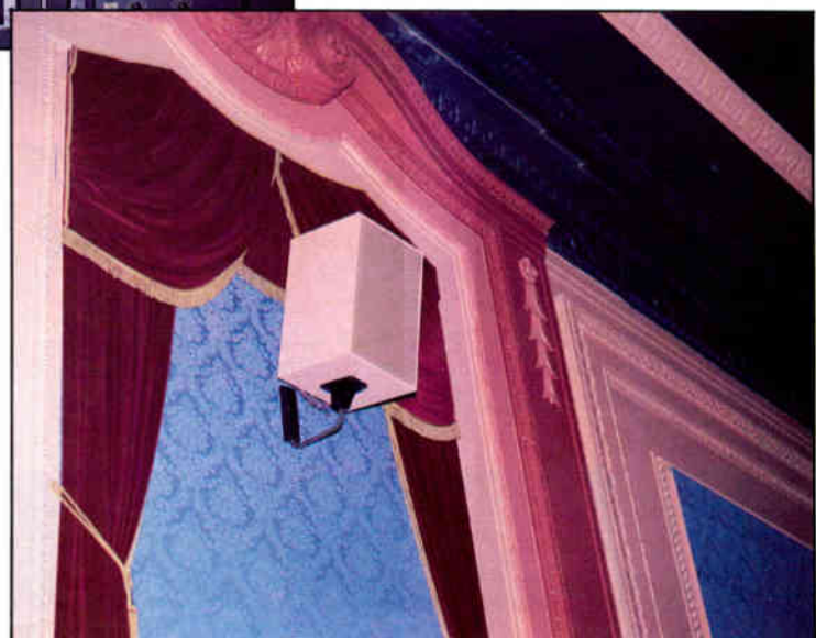
An SR-70 surround speaker installed at the Tivoli.
