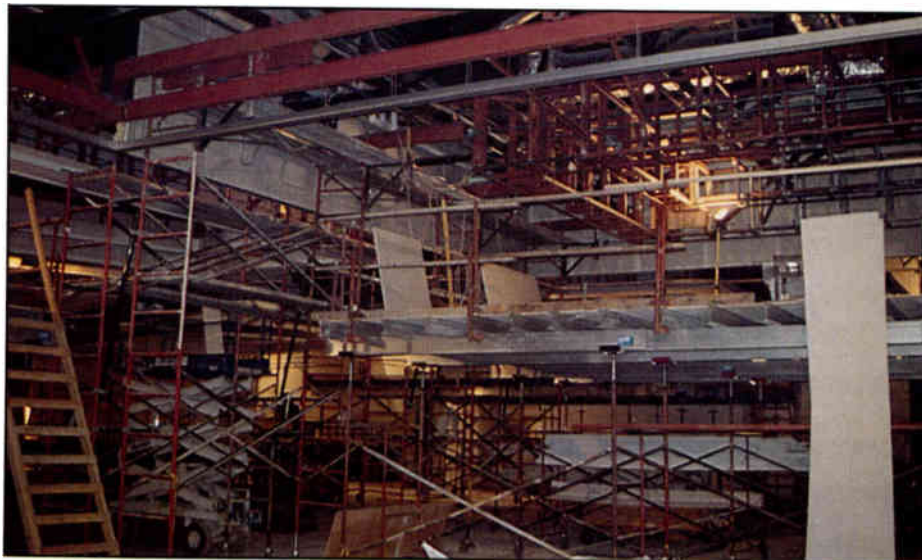
Colorado Hall construction phase.
