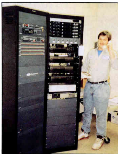
Installation at Butler County High School in Morgantown, Kentucky included a Rauland-Borg Telecenter IV Plus. Rick Williams from Comstar Systems in Bowling Green, Kentucky is shown.
