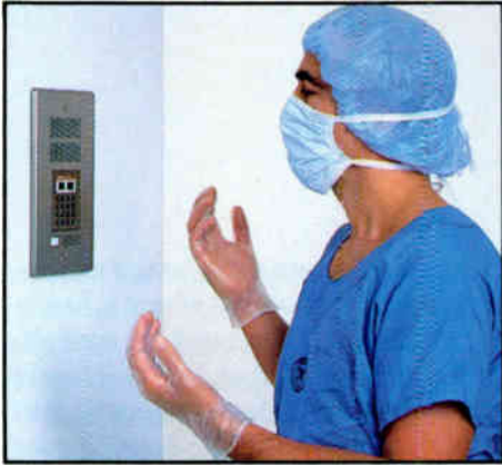
Aiphone installation at the UCLA Medical Center.
