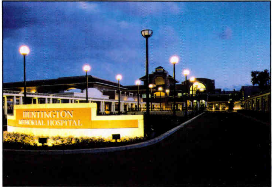
Huntington Memorial Hospital, California Building, Pasadena, California. Installation by Douglas Roesch Communications, Inc.
