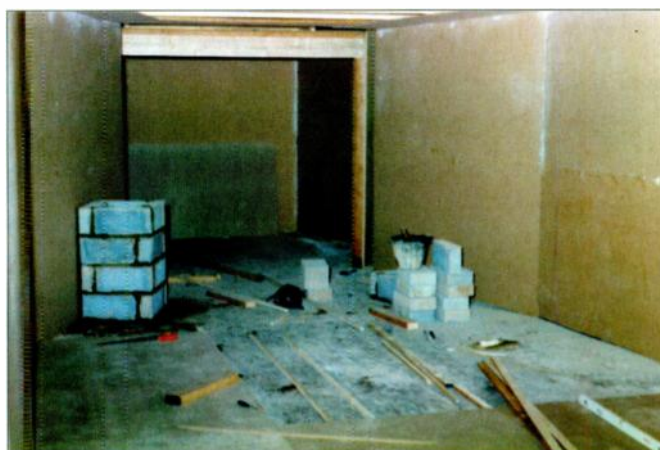
The Studio with inner shell walls in place.
