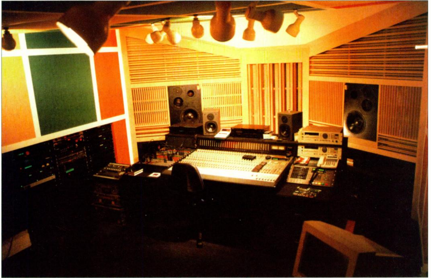
Martin Price (formerly of 808 State) commissioned the design of this room to produce the recent Kaliphx album. The simplified geometry of the room significantly reduced construction costs.
