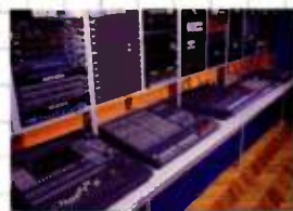
One side of the switcher-equipped recording room.
