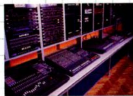
One side of the switcher-equipped recording room.
