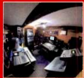
Dedicated room for studio monitoring
