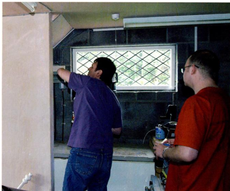
In an attempt to reduce the levels of bass leakage from the studio, Paul spent some time tapping various flat surfaces, such as underneath the stairs, to ascertain which ones were most likely to be resonating with the low frequencies.
