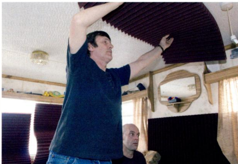
A few well-placed pieces of foam soon had the stereo imaging under control.
