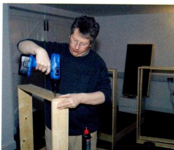
Hugh glues and screws the corners of the frames.
