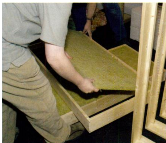
Fitting the rockwool slabs into the frames.
