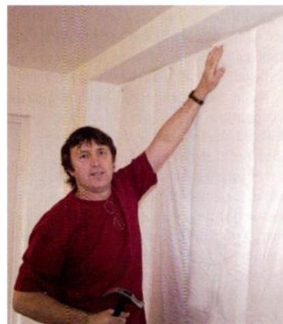
A return visit enabled Hugh and Paul to hang duvets in the recesses of the wooden garage doors, to further improve the room's acoustics.
