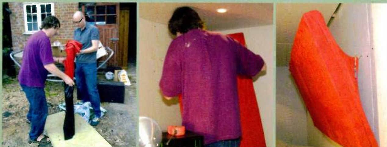
Some Ready Traps bags which Paul had brought with him allowed him and Simon to cover some Rockwool slabs and hang them from the studio walls from cup hooks as acoustic treatment.
