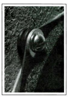
FIGURE I: An Audax 5½ driver mounts more easily with a rubber grommet. Notice the wrinkle finish paint on the baffle board.
