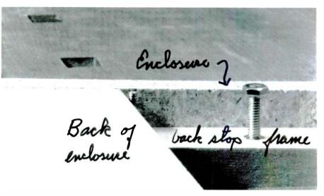
**PHOTO 13:** Relationship of the enclosure back, backstop frame, and the enclosure.
