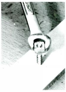
PHOTO 7: Installing a hanger bolt.
