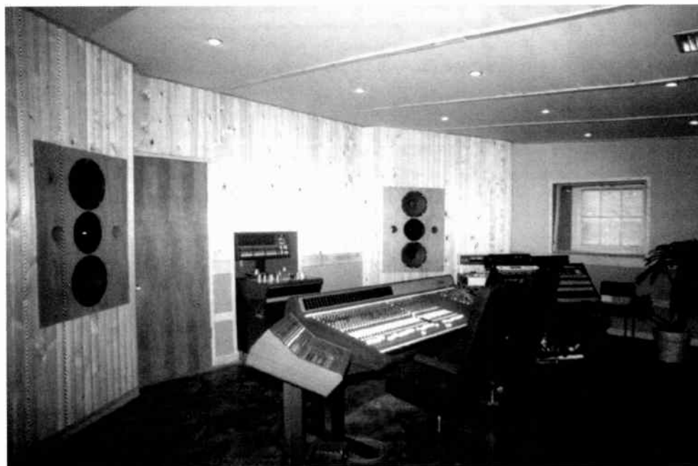
PHOTO 1: Recording studio constructed according to “nonenvironment room” principles.
