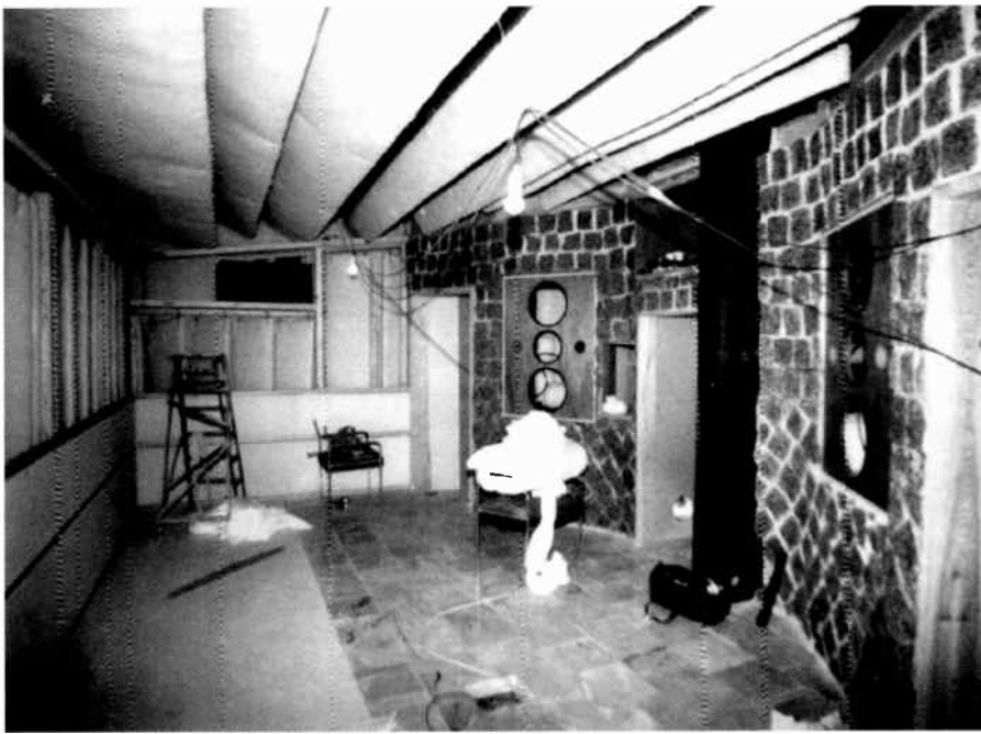
PHOTO 2: Building a nonenvironment room. Note accommodations for the monitor loudspeakers mounted flush in the front wall.
