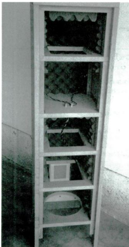
PHOTO 11: Foam and wiring installed in cabinet.
