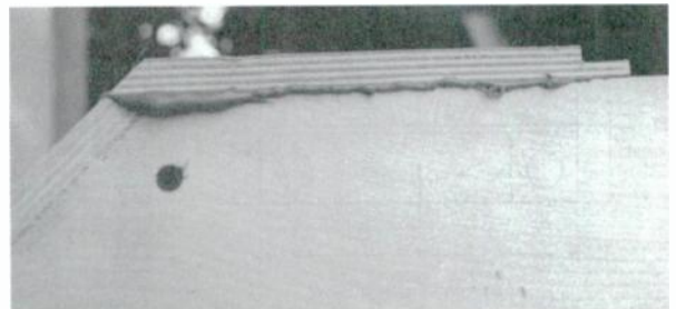
PHOTO 10: Detail of dado on cabinet's lower back.
