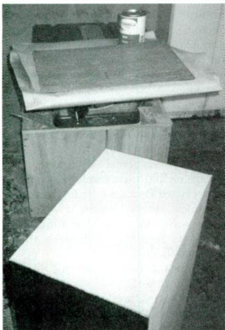
PHOTO 6: Formica panels cut oversized, with the adhesive allowed to dry before joining the cabinet and material together.
