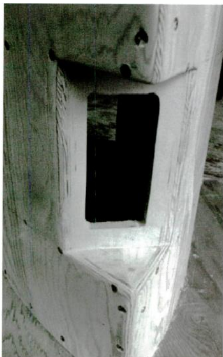
PHOTO 11: The completed horn assembly.
