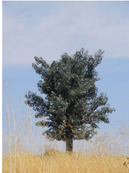
An SCI custom oak tree made for AT&T and placed at an antenna site in Sacramento, California.
