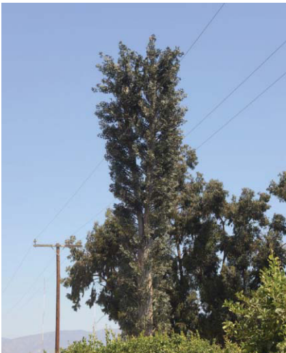
An SCI 100-foot multicarrier eucalyptus built for Verizon Wireless in Oxnard, California.
