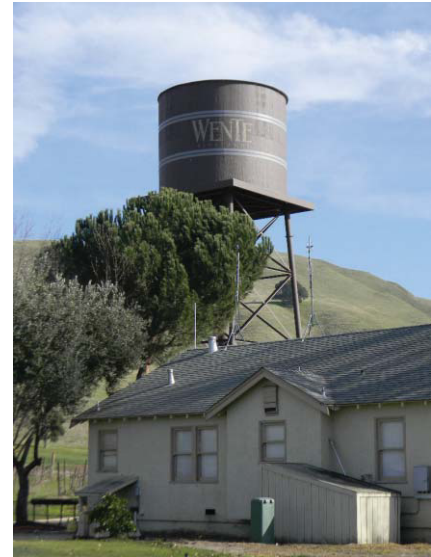
An SCI two-carrier, 75-foot water tank designed and built for AT&T to use in Livermore, California.
