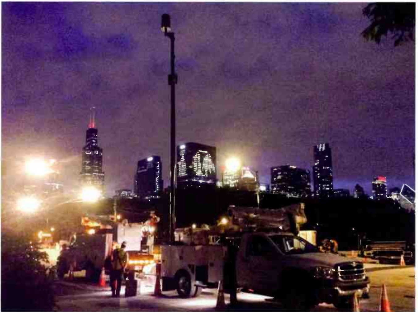
Installing light pole and small cell at night.
