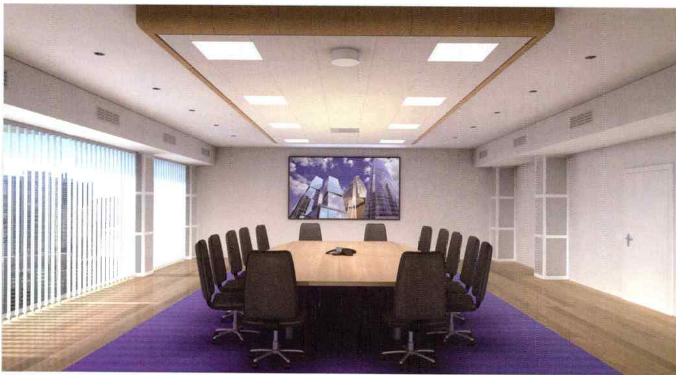
Shown on the ceiling in the foreground in a conference room, top and center in this image, a MIMO communications antenna draws little attention.
