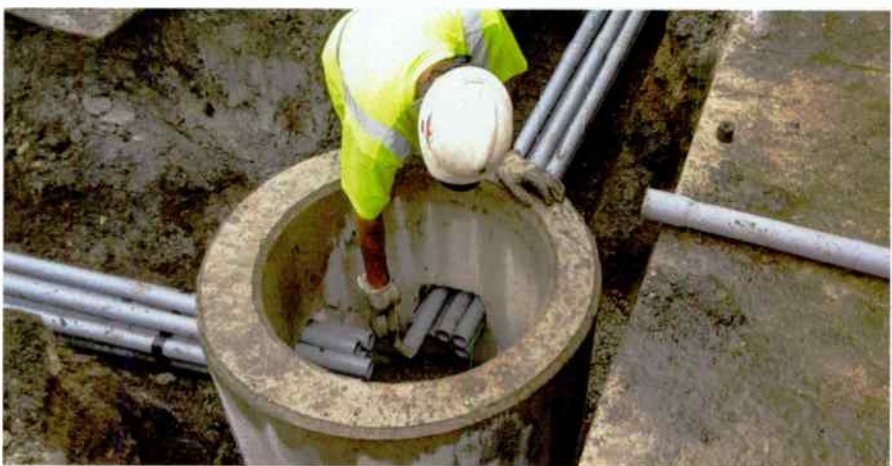
Finishing up the hand hole turn point.
