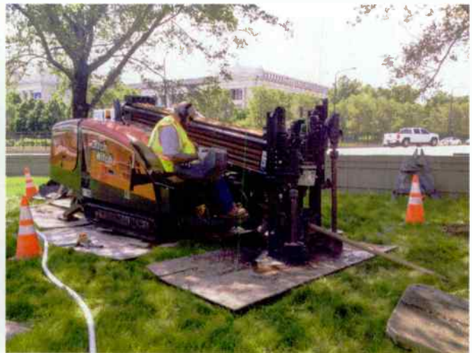
Left: Horizontal drilling 800 feet under sidewalk. Right: Drilling a 500-foot shot in Grant Park.
