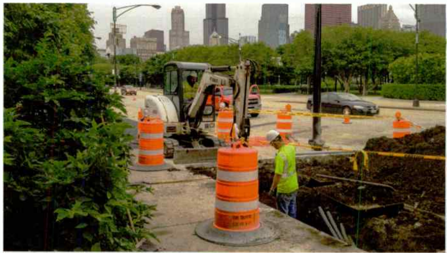
Excavating for a hand hole.
