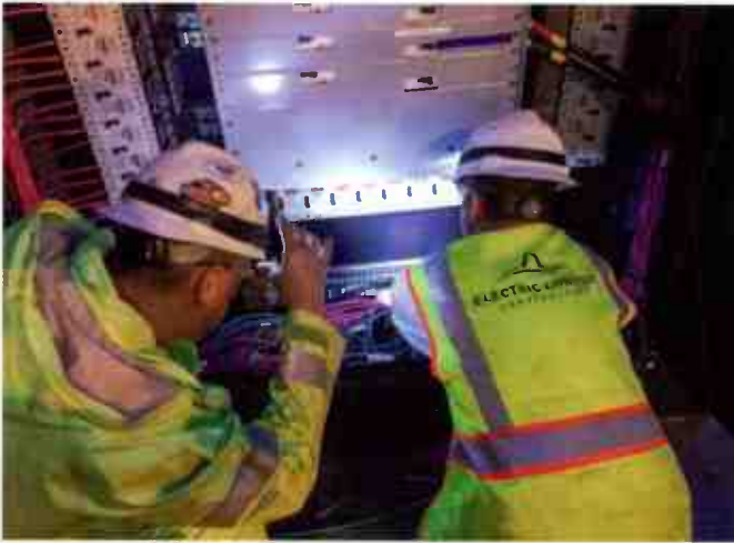
Left: Installing breakers and wiring power to small cell radio package. Right: Fiber-optic cable pulled through.
