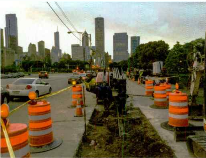
Left: Horizontal drilling 800 feet under sidewalk. Right: Drilling a 500-foot shot in Grant Park.
