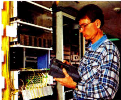
The MTS 5100 mini-OTDR is designed to handle single- and multimode installations.
