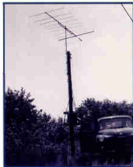
Early cable construction was a hit-and-miss proposition, as little training was available.
