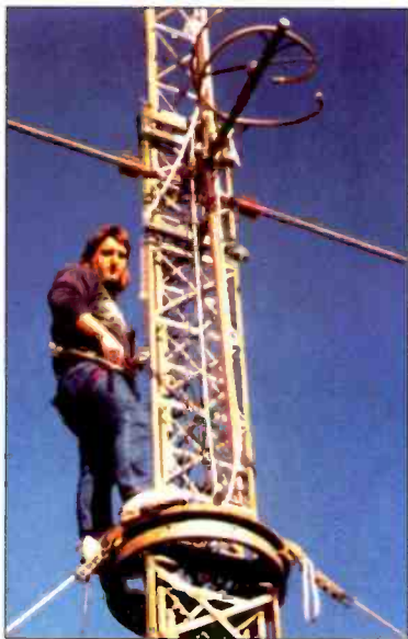
A circularly polarized antenna, such as this FMA-727 from Armstrong Transmitters, provides a signal in both the horizontal and vertical planes.
