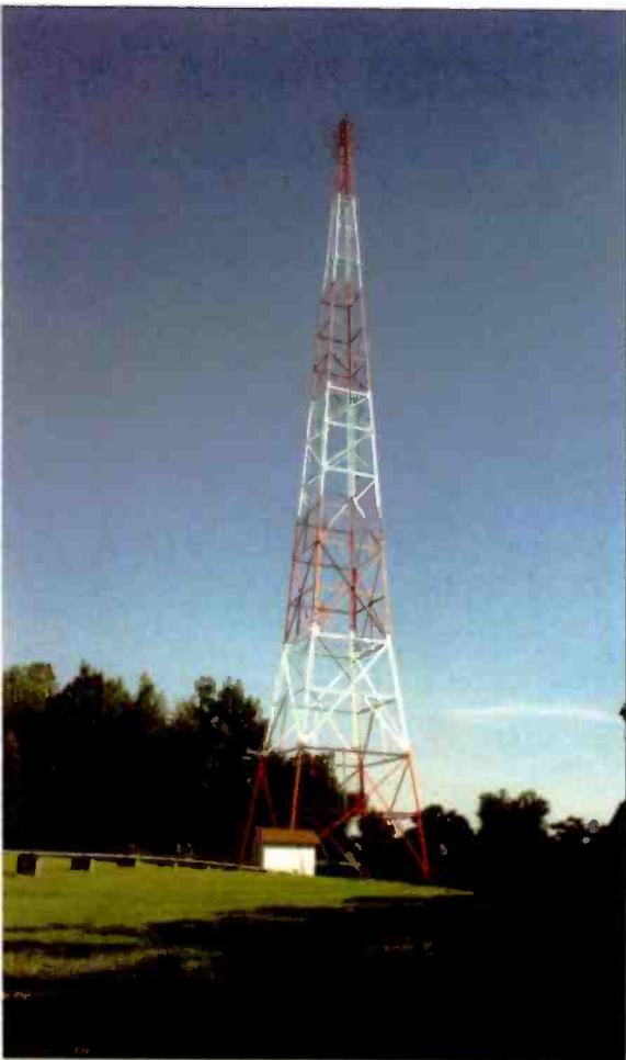
The locks on the doghouses resonate during the day when WAPI is at high power.
