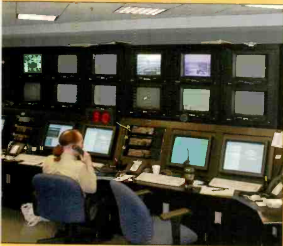
More than 50 terrestrial video cameras can be controlled by an operator at the video wall.
