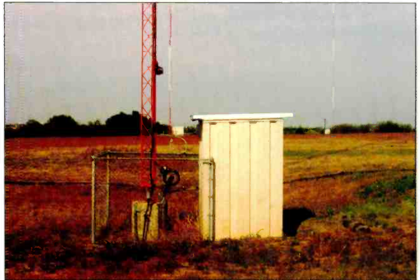
The base of tower eight and the original doghouse
