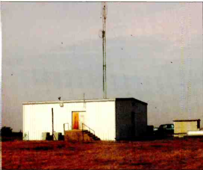
The stand-alone tower next to the transmitter building keeps the STL dish off the broadcast towers.
