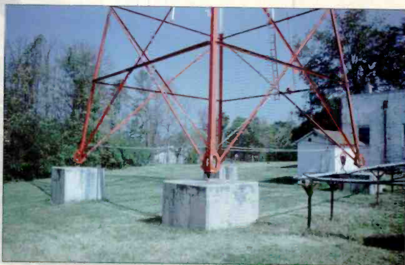
The neighbor's house where the singing washing machine lived is just beyond the transmitter site property line.
