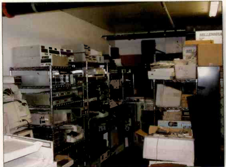
When multiple radio stations move in to the same facility, there is bound to be surplus equipment, making storage space a more important part of a facility design.
