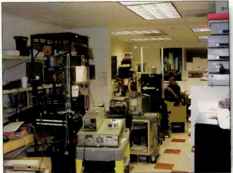
When consolidating multiple radio stations, plan an adequately sized engineering shop. In this facility, the chief engineer's office is next door.
