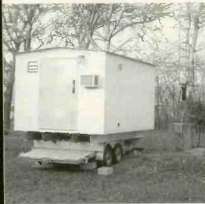
SCVS/WFAN Aux Tower New York, NY
