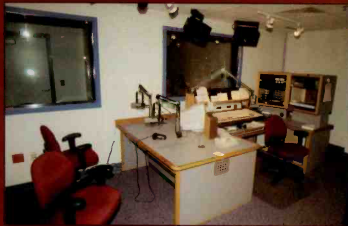
The On-Air Room uses a Harris Impulse-20 console.
