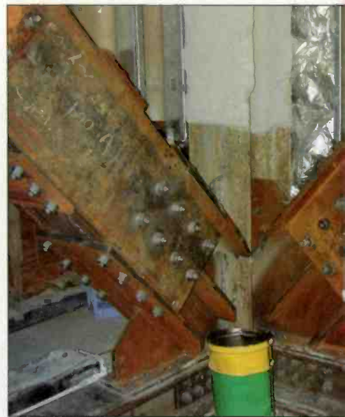
Additional steel reinforcements were needed to increase the structure's strength.
