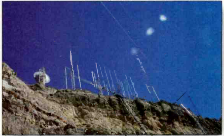
Looking up at the Apex Communications site, which serves as the middle point of the STL path.
