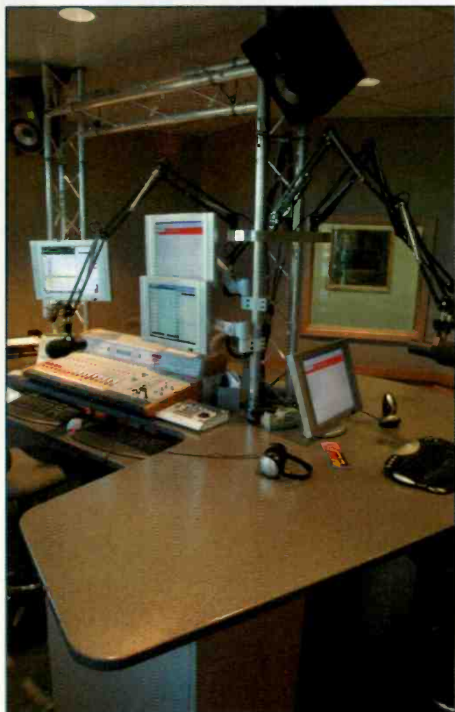
The air studios have similar layouts, and both use the trussing for a cable conduit and accessory mounting.
