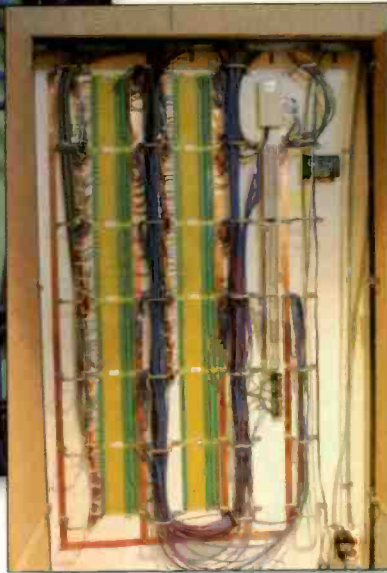
The Lindy blocks are used to terminate all the inter-studio wiring. The photo to the right shows the in-studio wiring closet in KFMA.
