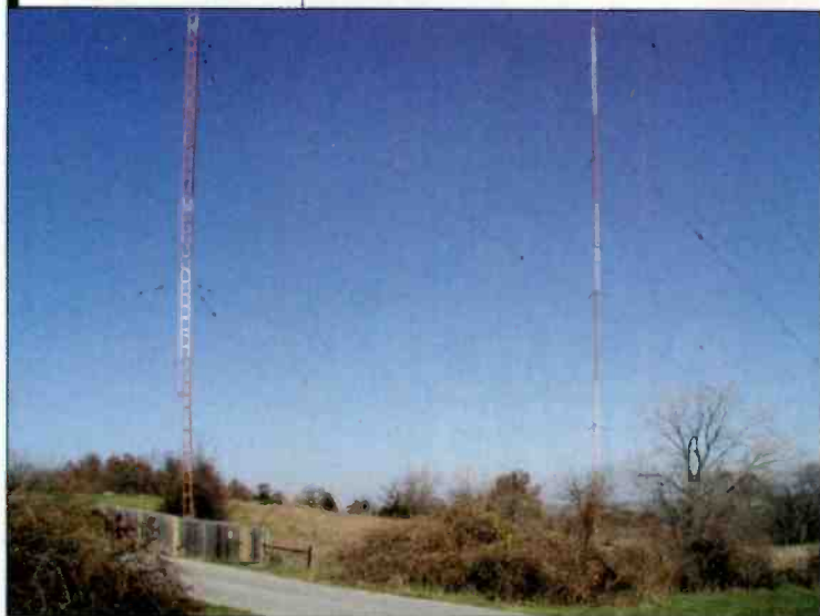
Physical changes in the antenna system can affect a directional array, but it is equally important to inspect tower fences and clear ground vegetation.
