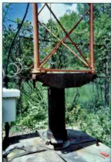
It is important to check the tower base insulator, spark gaps and tower feedline regularly.
