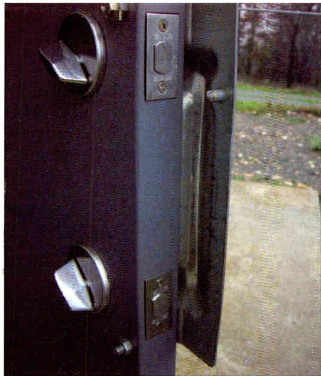
Figure 4. Bolted door locks with a cover slow the entry of an intruder.
