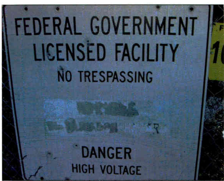
Figure 2. Signboards can warn trespassers of the severity of entering the station's premises.
