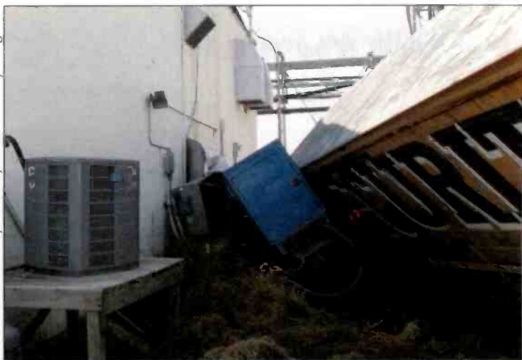
This generator was crushed by a storage van belonging to the CUU.
