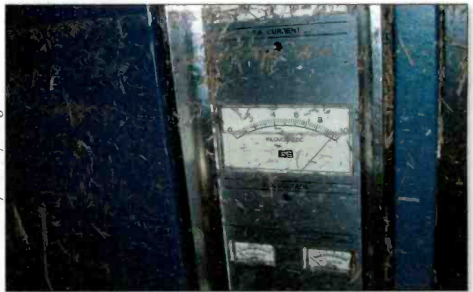
The transmitters for WRNO and WNOE-FM in New Orleans were flooded and left caked with mud and debris.
