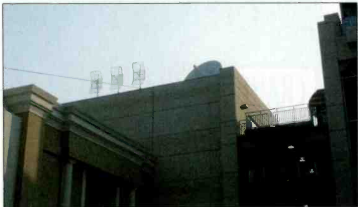
The STL and satellite antennas are mounted on the roof of the adjacent building.
