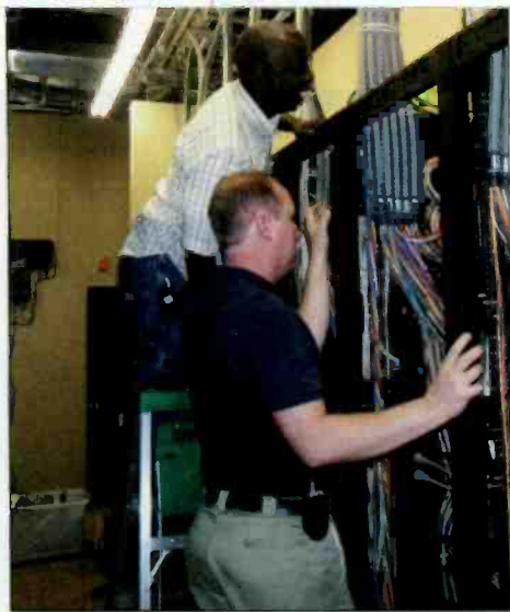
Hal Stinett and James Kester install rack equipment.
