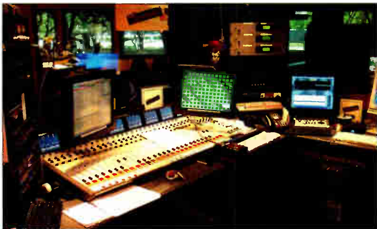
The TJMS control room is built around the Wheatstone G-9. The Vox Pro, Audio Vault, Stac and other auxiliary equipment are naturally within easy reach of the operator.
