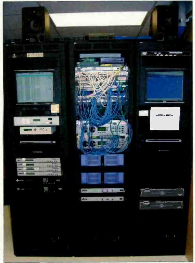
The engineering racks house the satellite receivers and Logitek and Enco servers.
