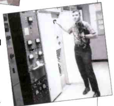
Burt at WOCB with the owner's (Wes Stidstone) dachshund. Pictured are a Gates 5kW transmitter and an RCA AM BTF1B (he believes) in the foreground. The RCA transmitters are 1kW and 250W (standby).
