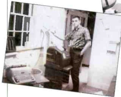
Burt at WOCB with the owner's (Wes Stidstone) dachshund. Pictured are a Gates 5kW transmitter and an RCA AM BTF1B (he believes) in the foreground. The RCA transmitters are 1kW and 250W (standby).
