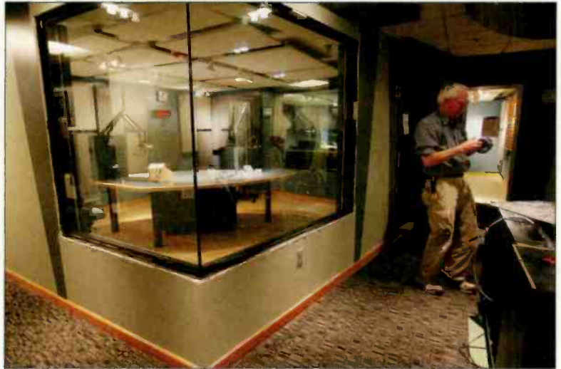
Studio B just as the final installation is nearly completed.
