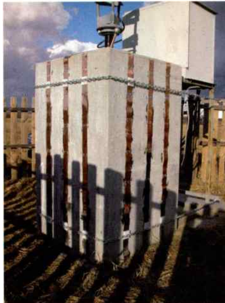
The owner of this site replaced the stolen ground strap on the pier, and then covered it all with a foundation cement.
