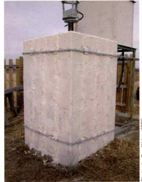
The owner of this site replaced the stolen ground strap on the pier, and then covered it all with a foundation cement.
