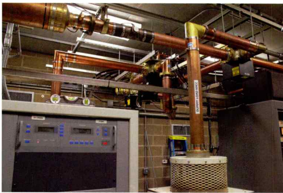
KHCC: RF plumbing that provides split-level combining in the ERI IBOX M-3 AND, with MCI 61304 switches, allows the station to bypass the combiner and put the Z16HD+ directly to air in any mode, FM or FM+HD for maintenance of HPX40. The old BE20B and HPX40 are also switchable.
