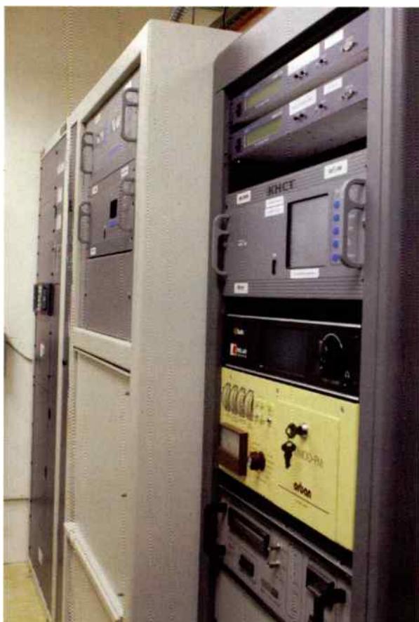
KHCC: RF plumbing that provides split-level combining in the ERI IBOX M-3 AND, with MCI 61304 switches, allows the station to bypass the combiner and put the Z16HD+ directly to air in any mode, FM or FM+HD for maintenance of HPX40. The old BE20B and HPX40 are also switchable.
