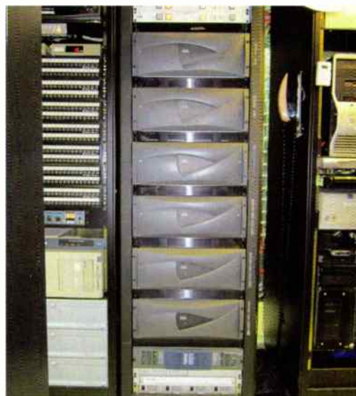
Multiple SAS 32KD frames (left) are integrated with a Harris D-series automation (center) and controlled by a workstation in master control (right).
