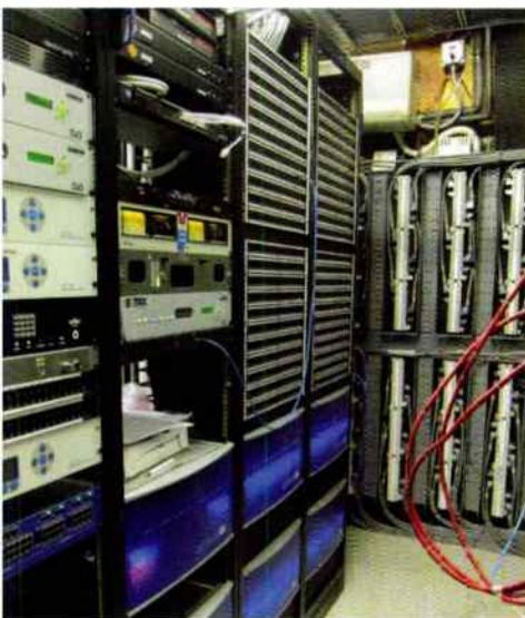
Multiple SAS 32KD frames (left) are integrated with a Harris D-series automation (center) and controlled by a workstation in master control (right).
