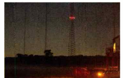
The KRKO/KKXA towers at night just prior to a test run
