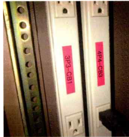
Figure 4: Redundant AC Power Feeds
